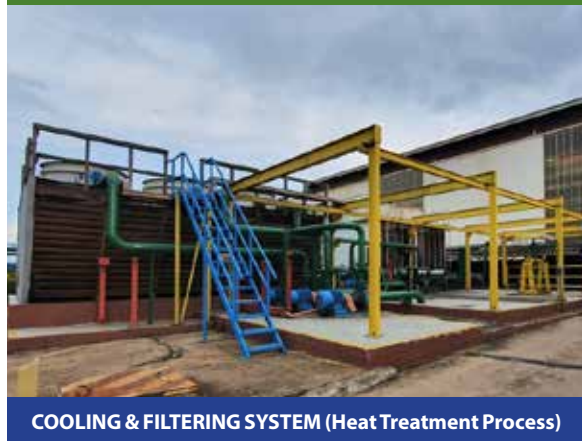
Implementation Close Loop System to re-use waste water from Heat Treatment & NDT process
