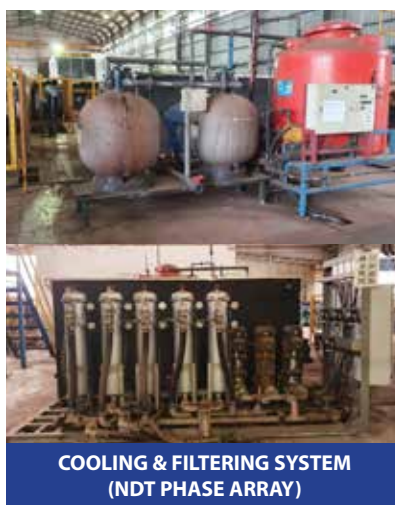
Implementation Close Loop System to re-use waste water from Heat Treatment & NDT process
